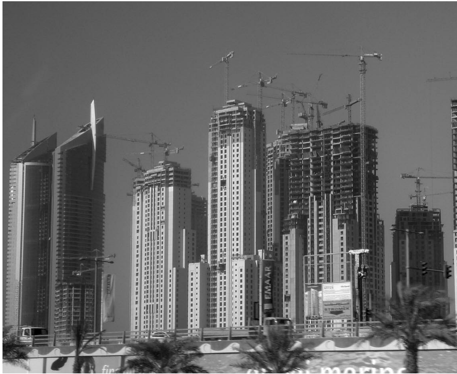
Construction site, Dubai.
